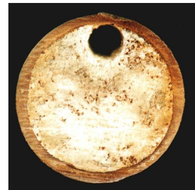
Water scale in a pipe
